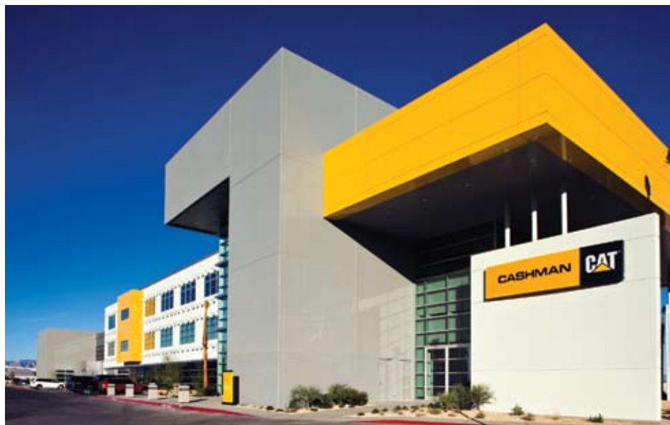
Cashman Equipment Co.'s new headquarters is located at 3300 St. Rose Parkway.
