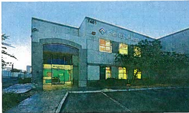
K2 Energy started out in a 200-square-foot space in the Henderson Business Resource Center. Within a year's time, the lithium battery manufacturer launched its first product lines. It recently opened a new 20,000-square-foot industrial space.
